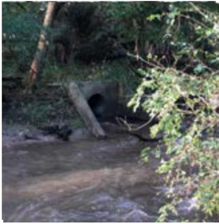
Chlorinated and saltwater can directly enter nearby streams if discharged into a storm sewer intake (ISWEP)
