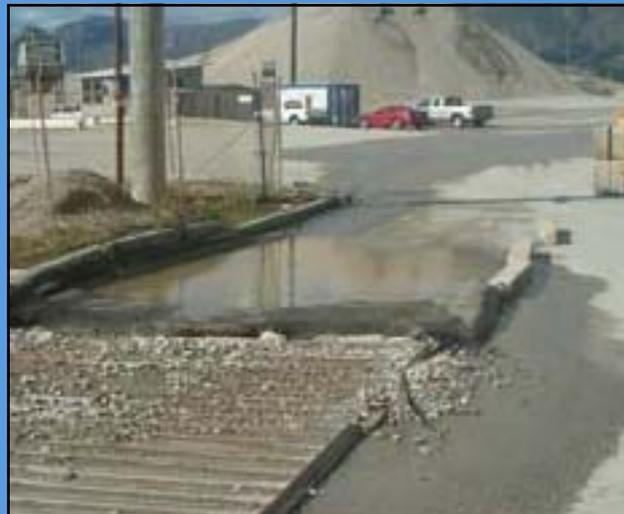
**Wash basin used for wheel washing. Note the rumble gate for added tire agitation and rock** (Mark Kestner).
