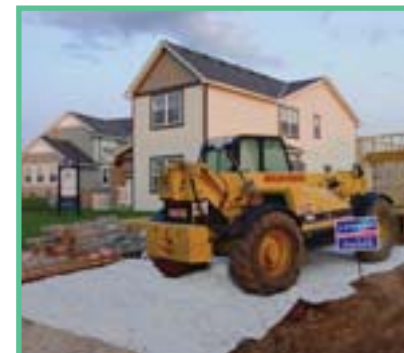
Stabilized exit at home site.
