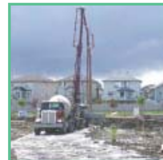
Stabilized construction exit.
