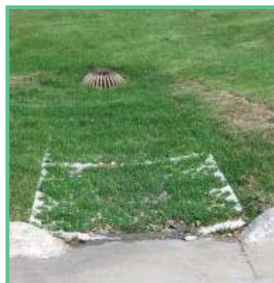
Stormwater flow from parking lot stabilized and vegetated with flow mats.
