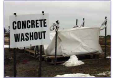
This designated concrete washout keeps pollutants from entering inlets and surface water.
